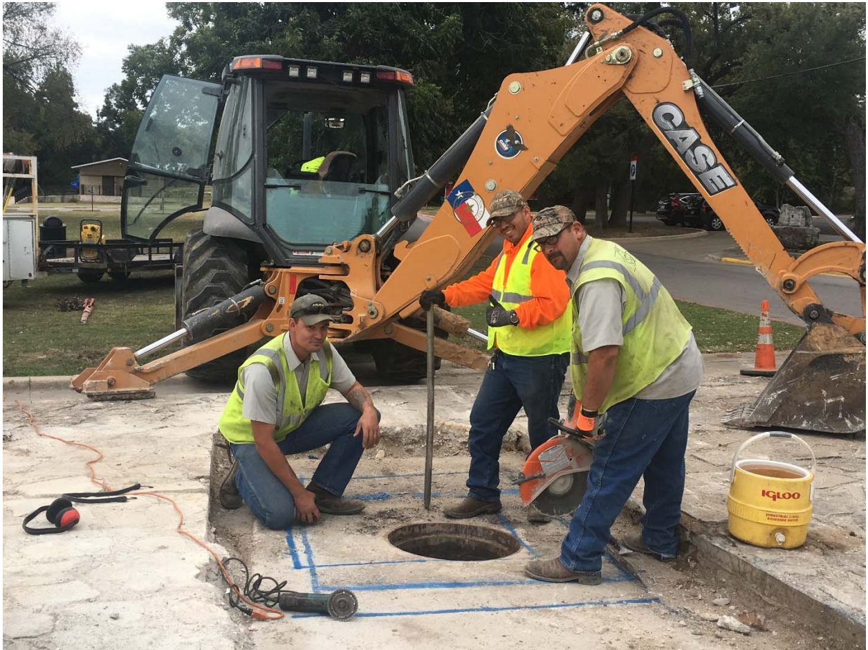
Sewer manhole repair, Fall 2017.
