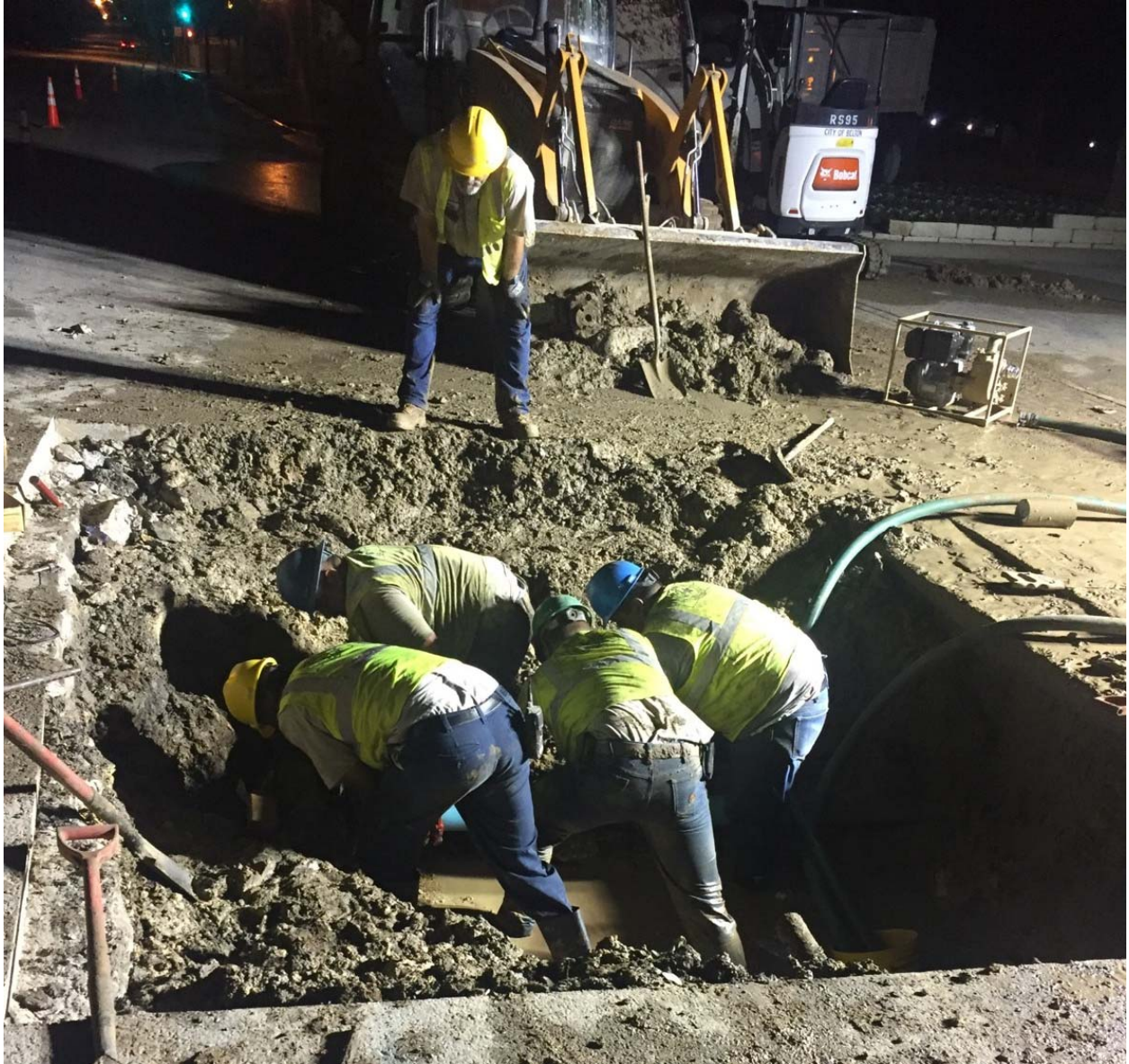
Waterline repair, Summer 2017.
