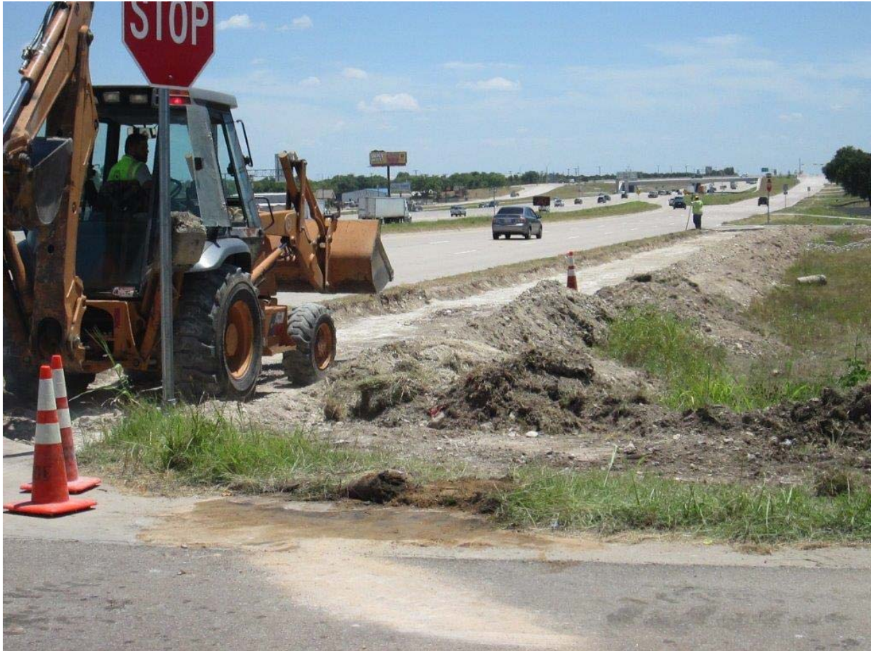
Sidewalk construction. Interstate Highway 35, Summer 2017.
