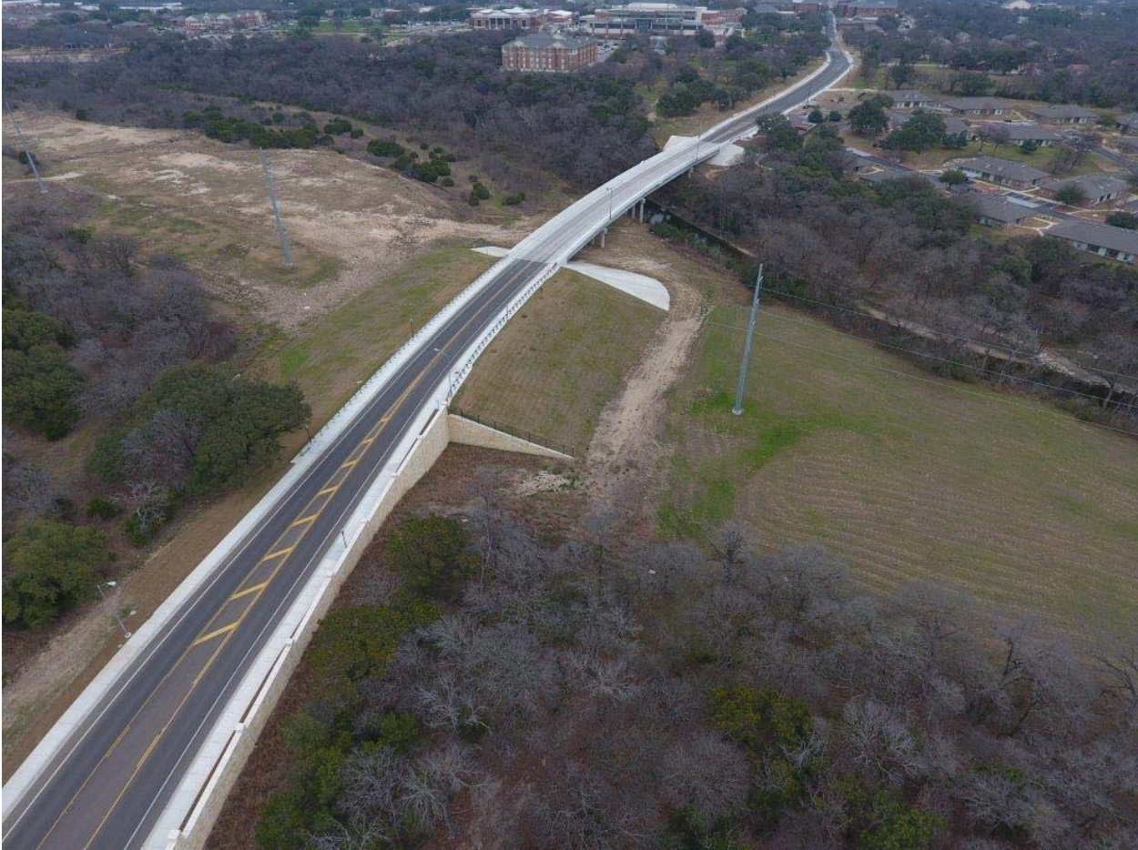
Martin Luther King Jr. Avenue Bridge, Winter 2016.
